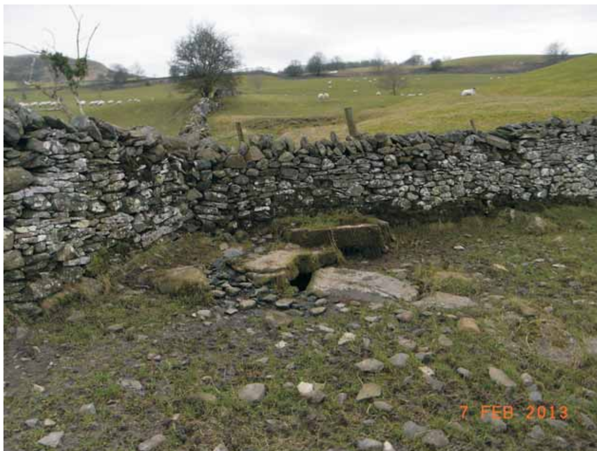
Plate 5: Spring and culvert
