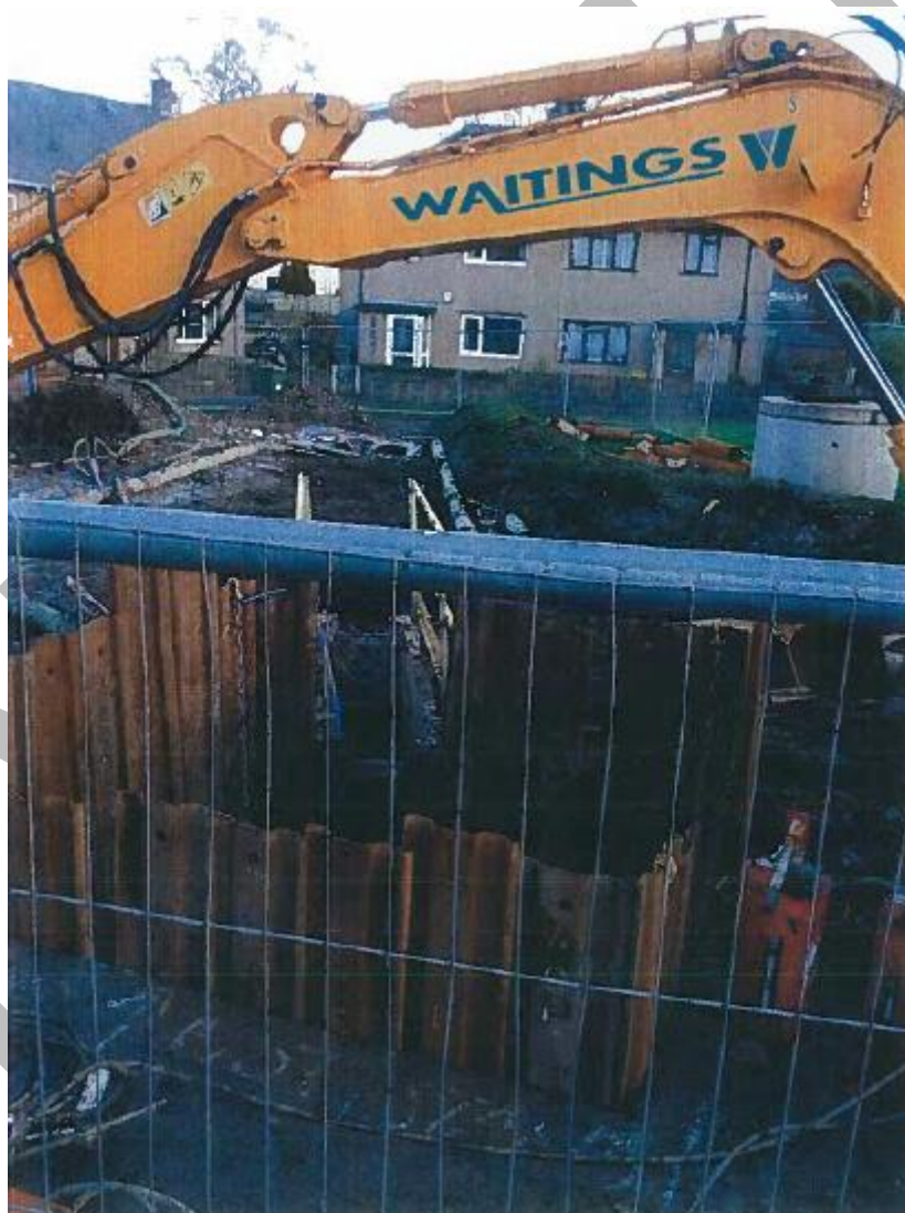
Works to repair drain Low Garth Photograph provided by United Utilities
